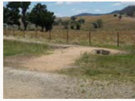
The existing walking track lacks shade and has areas of poor drainage.
