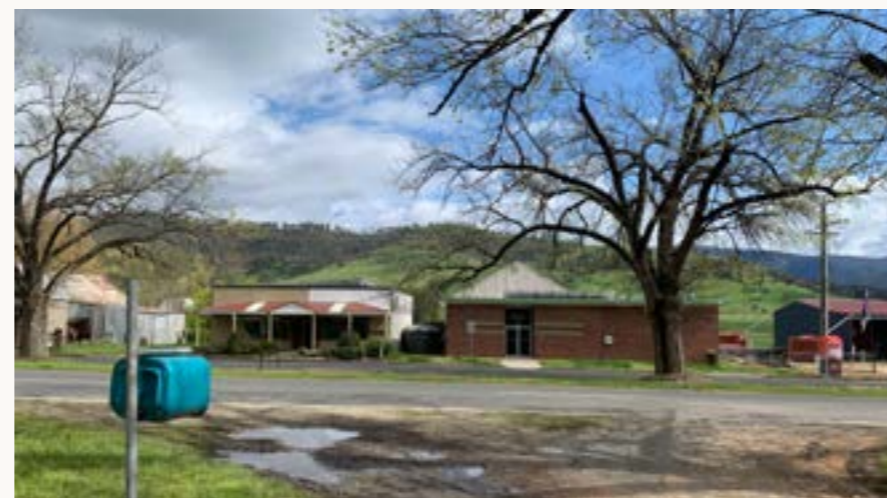
Parking is undefined in front of the hall and playground. Provide sealed designated car parks with signage for bus stop.
