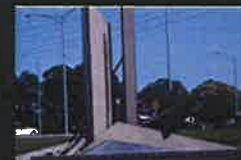
New central town entrance to clearly define town's street. (Oshana, Eastern Namibia, South Africa)
