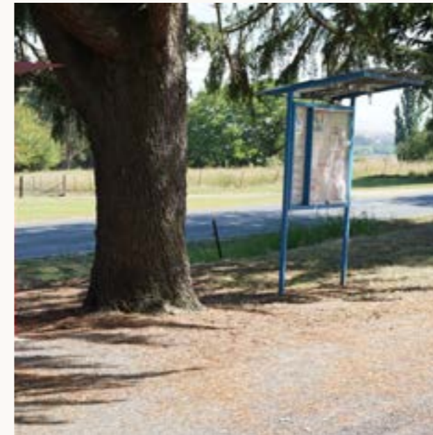
Community noticeboard requires replacement.
