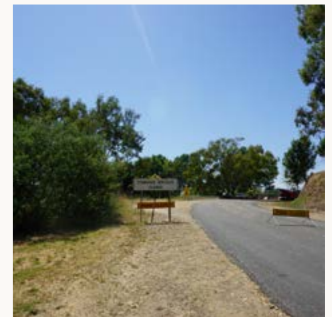
A pedestrian link between the beach area and the new bridge is required.
