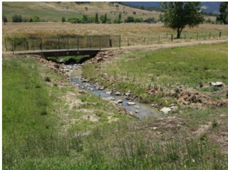
Poor drainage has impacted accessibility.
