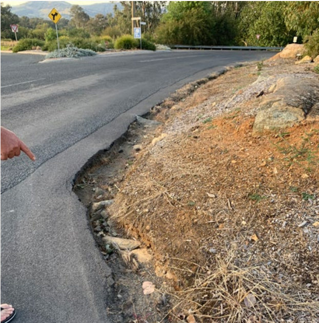
Damaged asphalt road surface on the south east approach to the bridge
