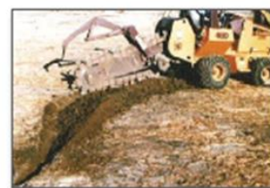
Figure 15. Trenchers make a wider excavation at turns
