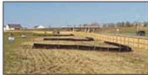
Figure 5. Use J-hook fences to break up long fence runs
