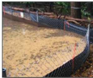
Figure 11. Chain link supported silt fence
