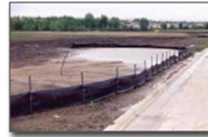
Figure 10. Gentle slopes may require a silt fence
