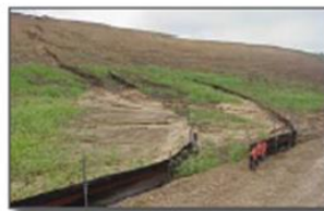
Figure 23. New silt fence below the old fence
