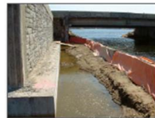
Figure 19. Silt fence for bridge abutment excavation
