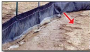
Figure 16. Poor compaction has resulted in infiltration and water flowing under this silt fence causing retained sediment washout
