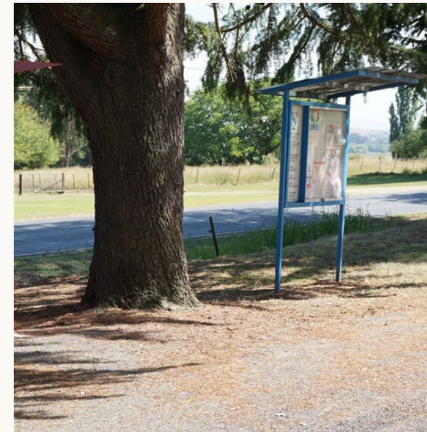
Community noticeboard requires replacement.
