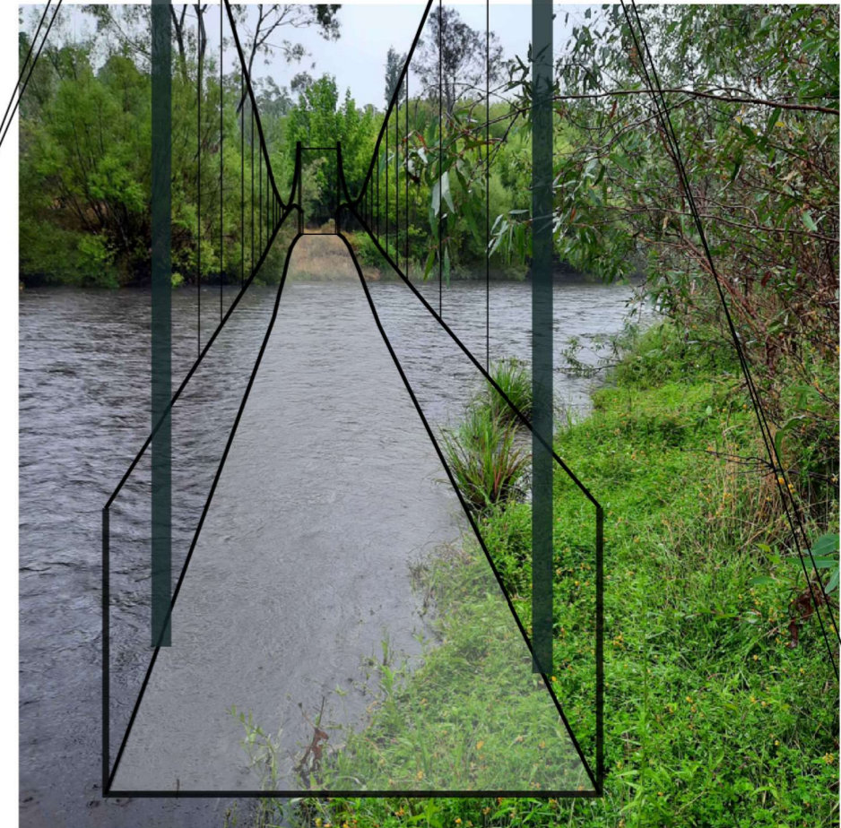
SUSPENSION BRIDGE - MITTA RIVER CROSSING (LOOKING AT EASTERN BANK)
