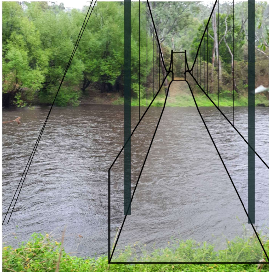
SUSPENSION BRIDGE - MITTA RIVER CROSSING (LOOKING AT WESTERN BANK)
