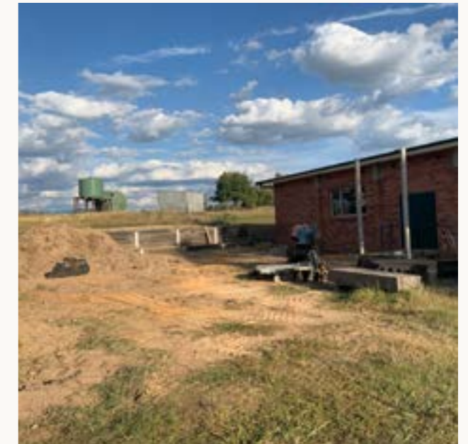
New event space and hall entry in construction
