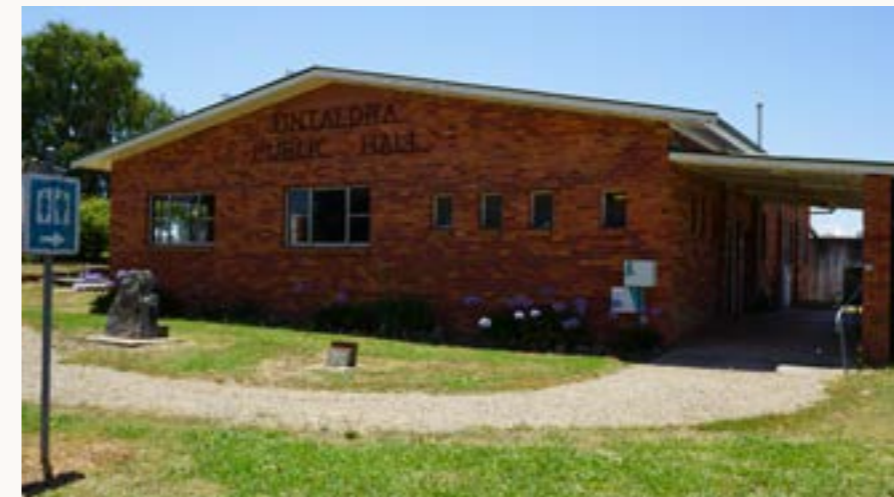
Public toilets are located in the Hall and can be difficult to find and access.
