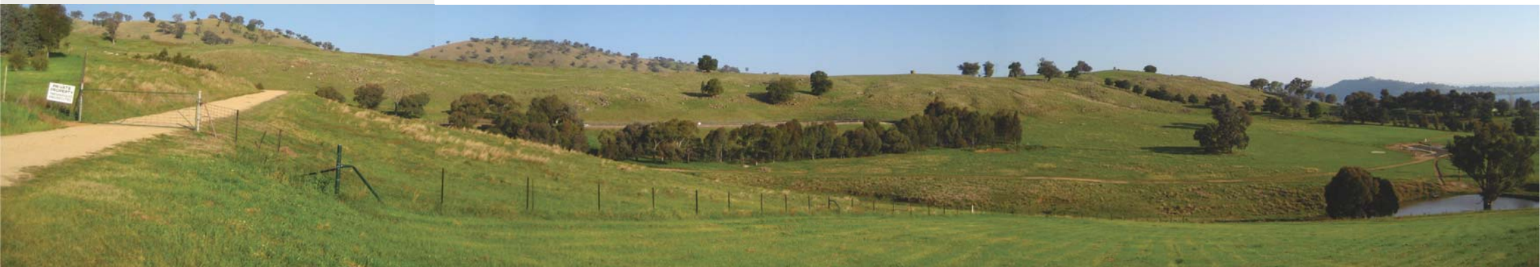
Sewerage Treatment Works
