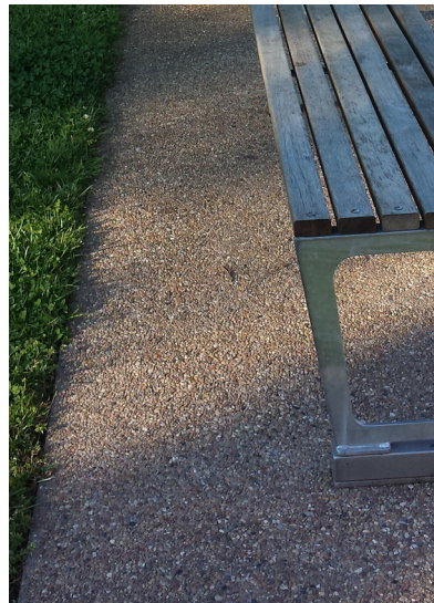
Hard sealed surface - concrete aggregate
