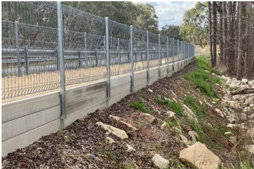
Retaining wall treatment on M2M Rail Trail
