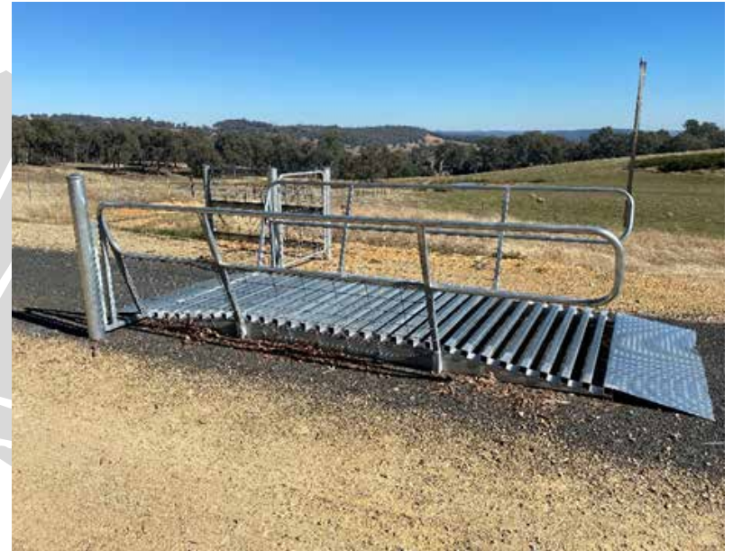
Farm crossing gateway, cattle grid solution, Tumbarumba
