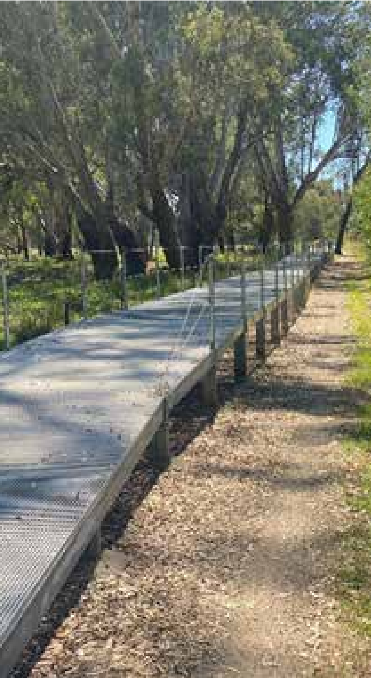
Elevated platform at Finn Creek
