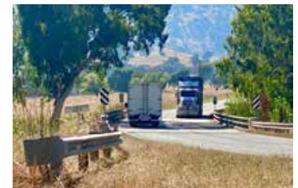
Tallangatta Creek Rd diversion
