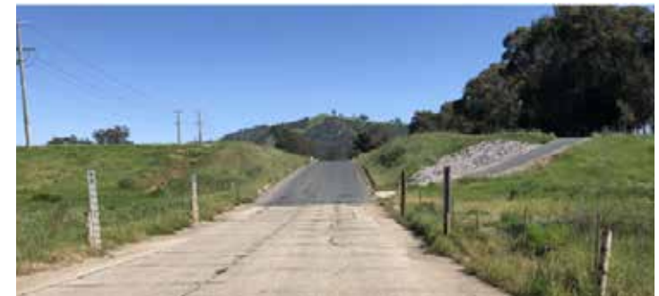
Whytes Rd Spillway
