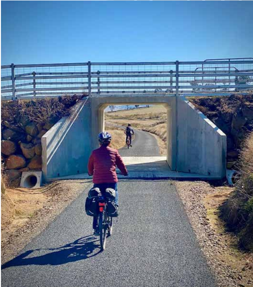
Farm crossing overpass, Tumbarumba
