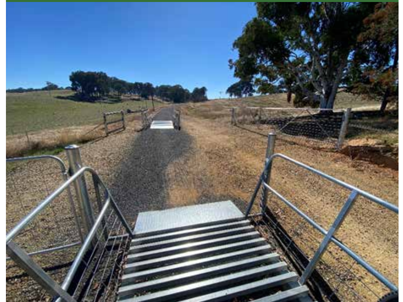
Farm crossing gateway, cattle grid solution, Tumbarumba
