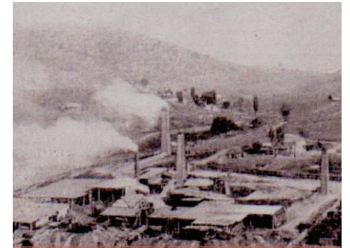
Wallace Bethanga Chlorination Works, circa 1897
